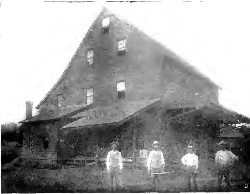
OLD VANDALIA FLOURING MILL.
